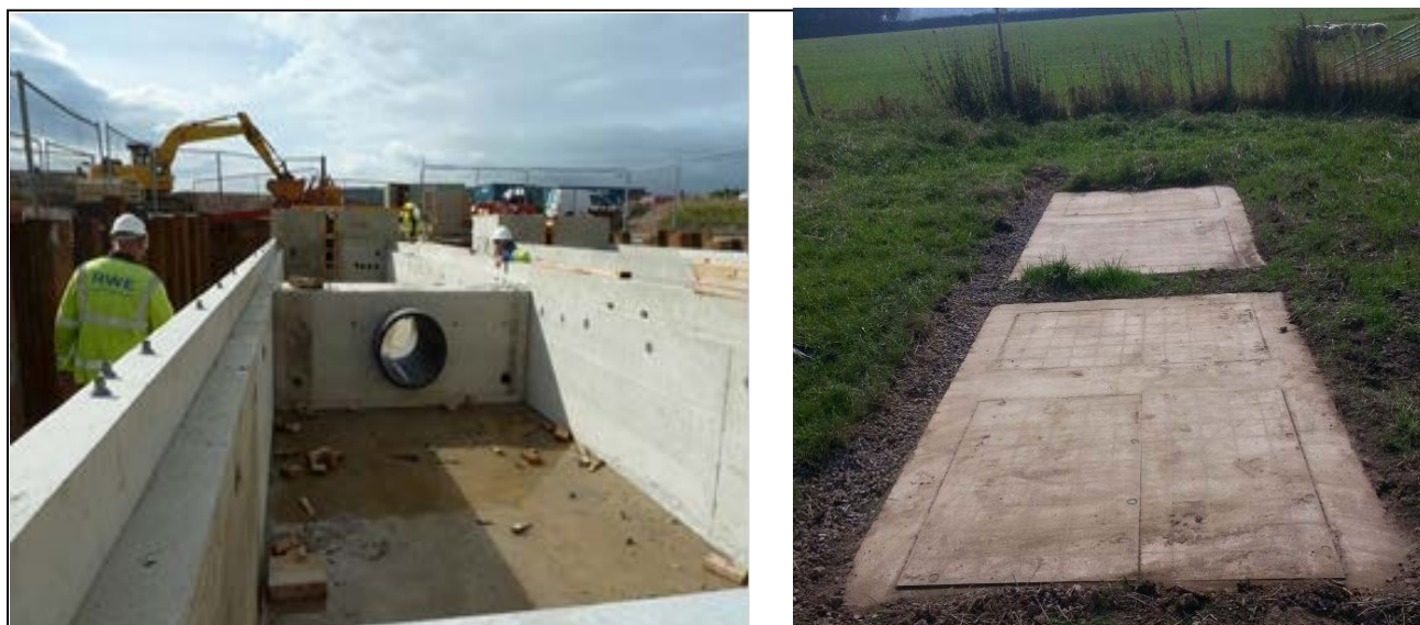
Figure 1.20: Typical TJB during construction (left) and after reinstatement (right)
